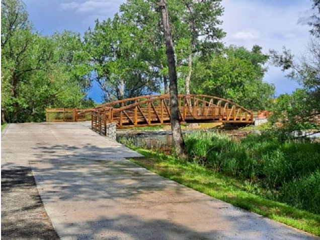
Accessible greenways such as the Bear Creek Trail promote a balance between urban infrastructure, open space, and the natural environment.
