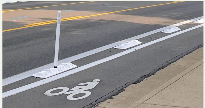
Figure 23: Plastic curbs and posts provide a relatively low-cost separated bike lane on Garrison St.
