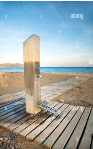
Foot Washing Station
