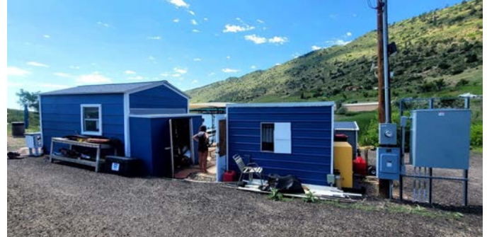
Existing Condition of Little Soda Lake Exterior
