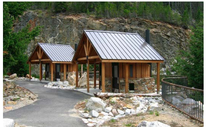
Example Image of Vault Toilet
