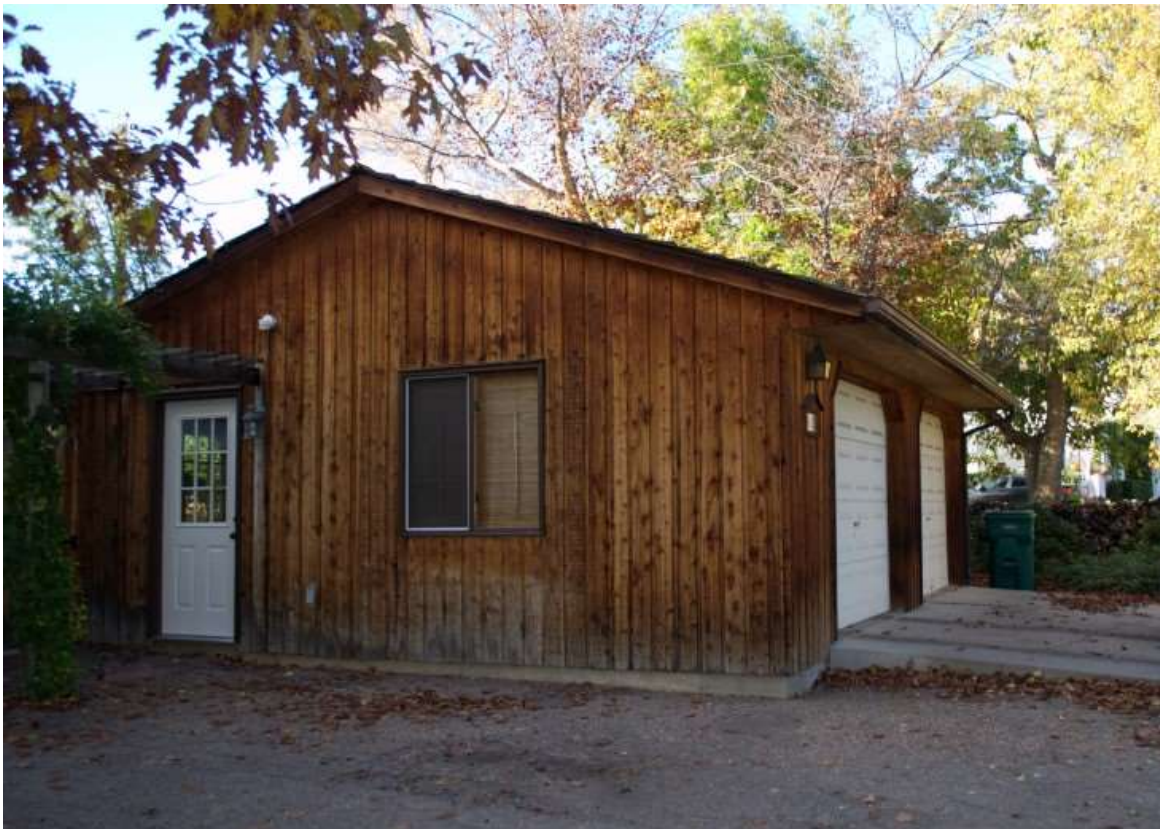
South-facing side of ca. 1995 two-car detached garage, looking north
