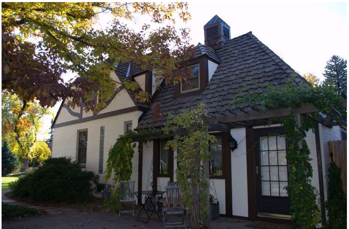
East-facing side of main section (left) and original garage (right), looking southwest
