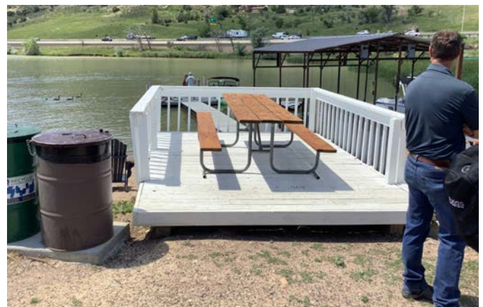
Existing Deck Proposed To Be Removed
