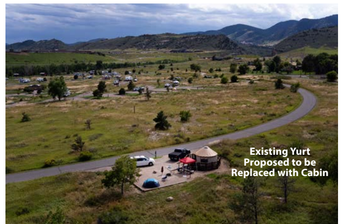
Existing View of Campground Looking South
