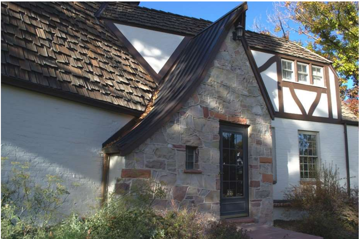
Cut stone-faced main entrance with copper clad catslide roof on main (southeast) façade, main section, looking northeast
