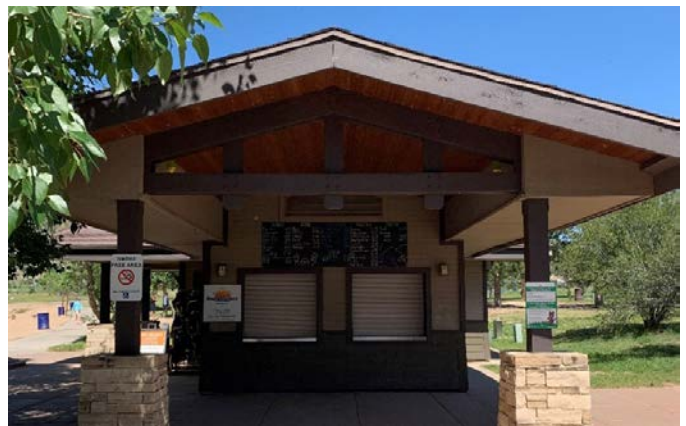
Existing Condition of Food Concessions Exterior
