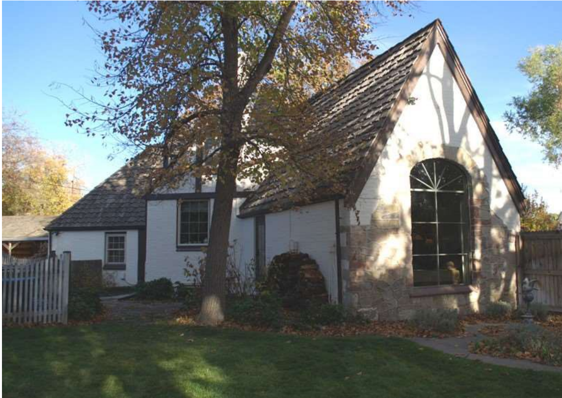
Photo: West-facing side – main section in middle and southwest wing on right
