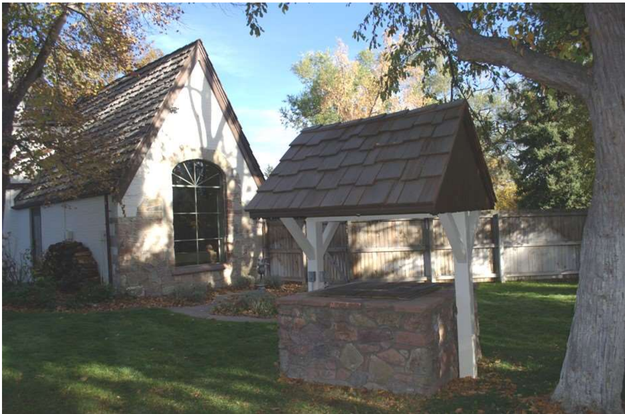
Well structure, west of the southwest wing (in background), looking southeast
