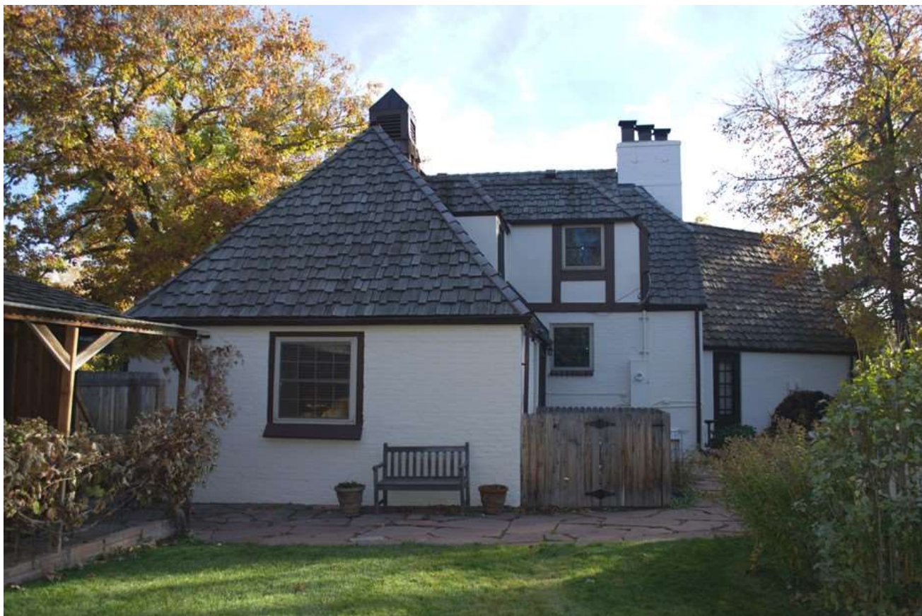
North-facing side – original garage (on left), main section (middle) and southwest wing with rear entrance (on right) looking south
