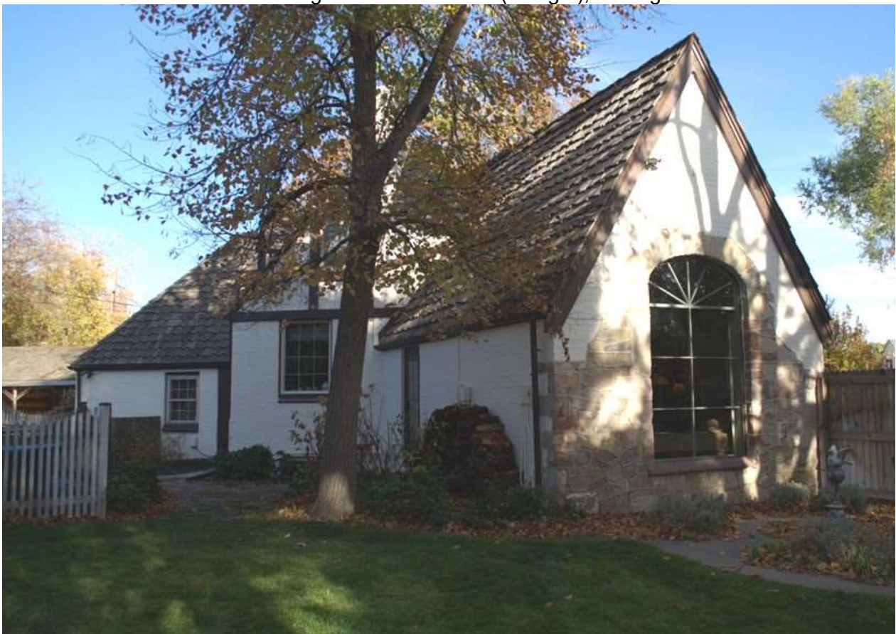
West/northwest-facing side – original garage (on left), main section (in middle), and southwest wing with rear entrance (on right), looking southeast
