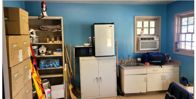
Existing Condition of Ranger Station Interior
