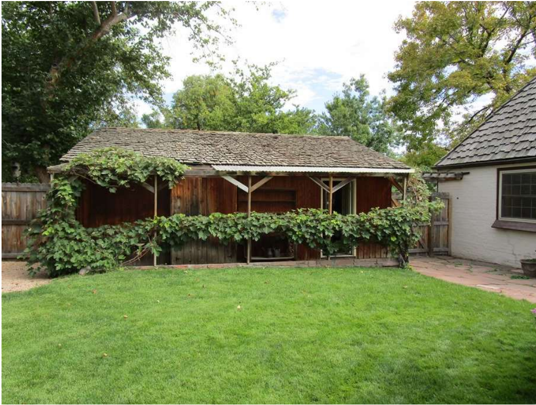
West-facing side of ca. 1995 two-car detached garage, looking east
