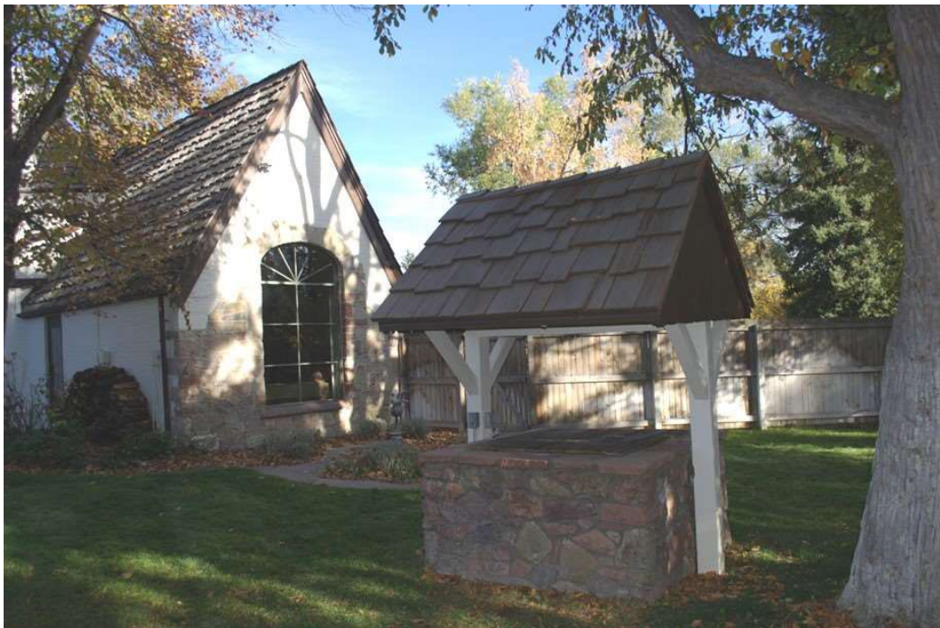
Photo: Close up of west-facing side with cut stone-faced window surround and well structure
