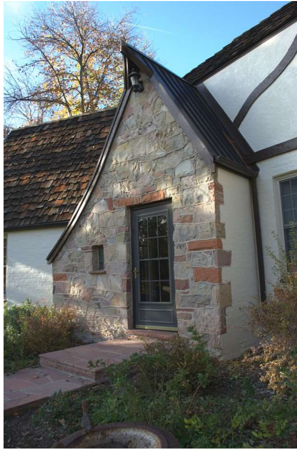
Cut stone-faced main entrance with copper clad catslide roof on main (southeast) façade, looking northwest
