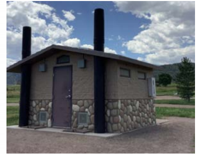
Example Image of Vault Toilet
