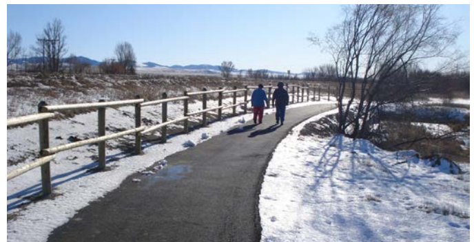
Example Image of Paved Trail
