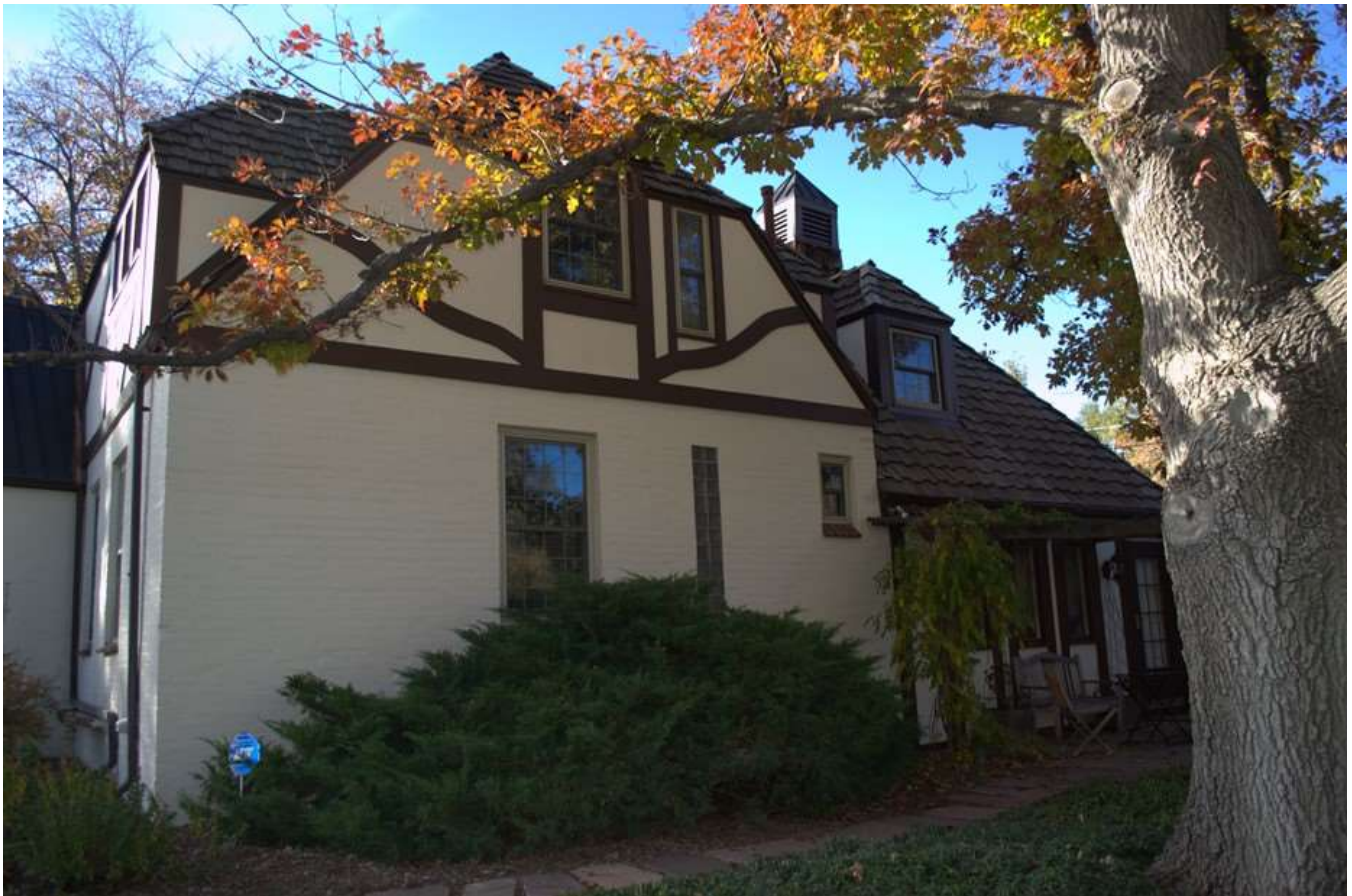
East-facing side of main section (left) and original garage (right), looking northwest
