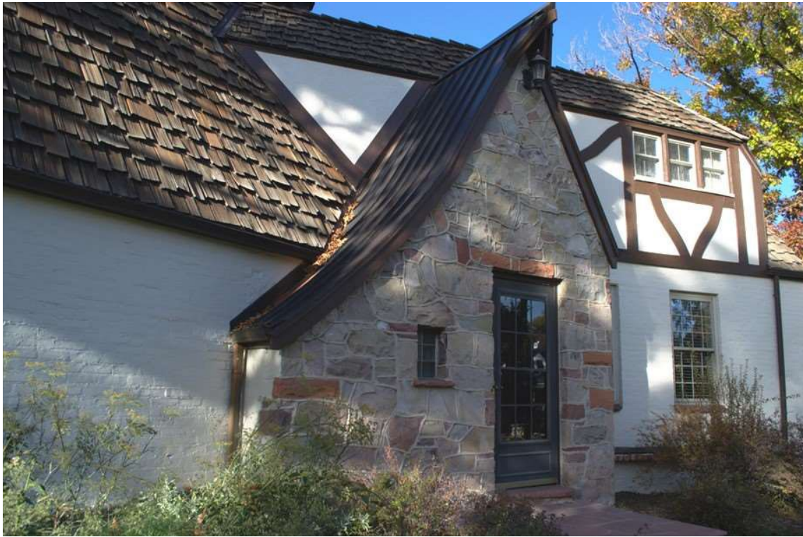
Photo: Detail of front elevation with cut stone entrance and copper clad catslide roof
