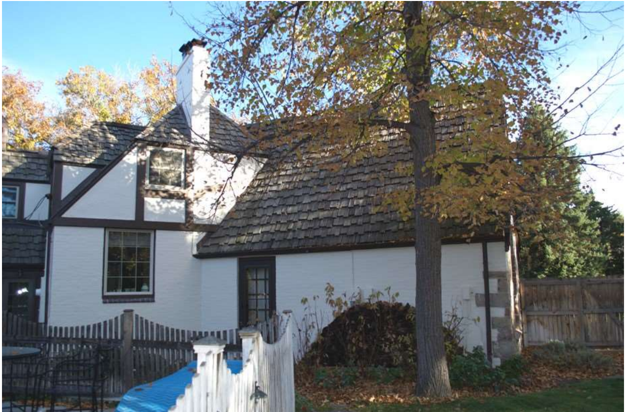
West/northwest-facing side – portion of original garage (on left), main section (in middle) and southwest wing with rear entrance (on right), looking southeast
