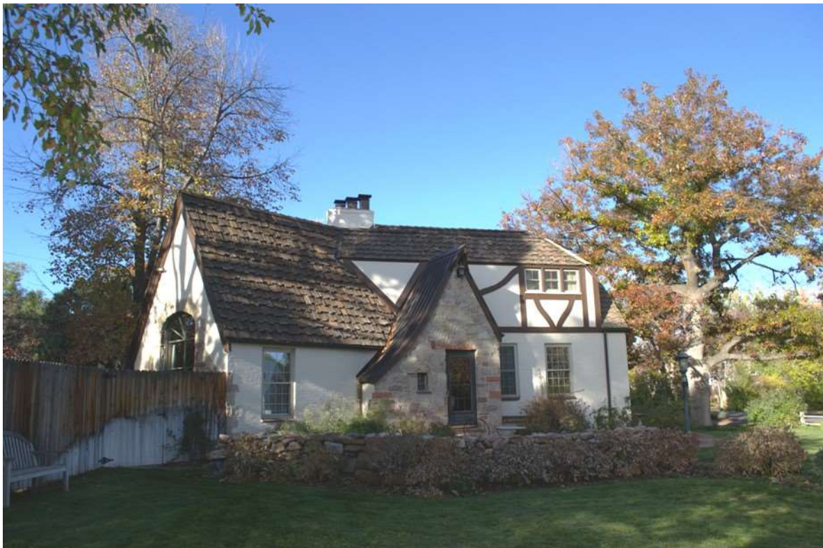
House with stacked stone retaining wall, looking northeast
