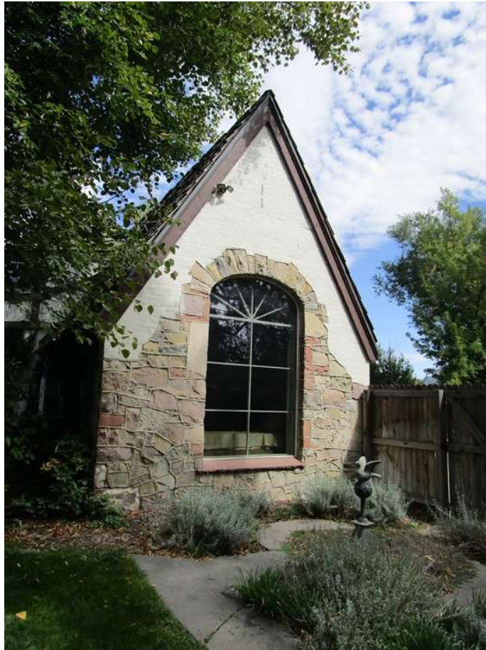
Close up of southwest wing, southwest-facing side, with cut stone-faced window surround, looking southeast
