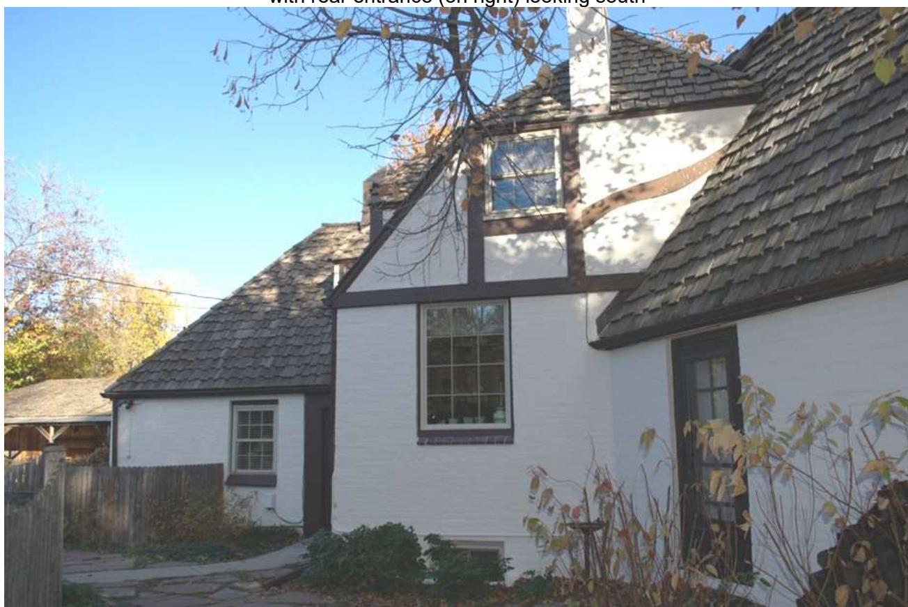
West-facing side –original garage (on left), main section (in middle) and southwest wing with rear entrance (on right), looking east
