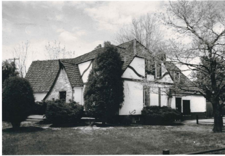
Ca. 1990 photo of the Miller House, showing rock-faced entrance, camera facing northwest. Unknown photographer. Courtesy of Heritage Lakewood Belmar Park.
