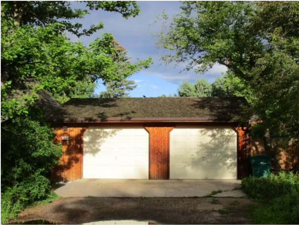
East-facing side of ca. 1995 two-car detached garage, facing Glen Dale Drive, looking west
