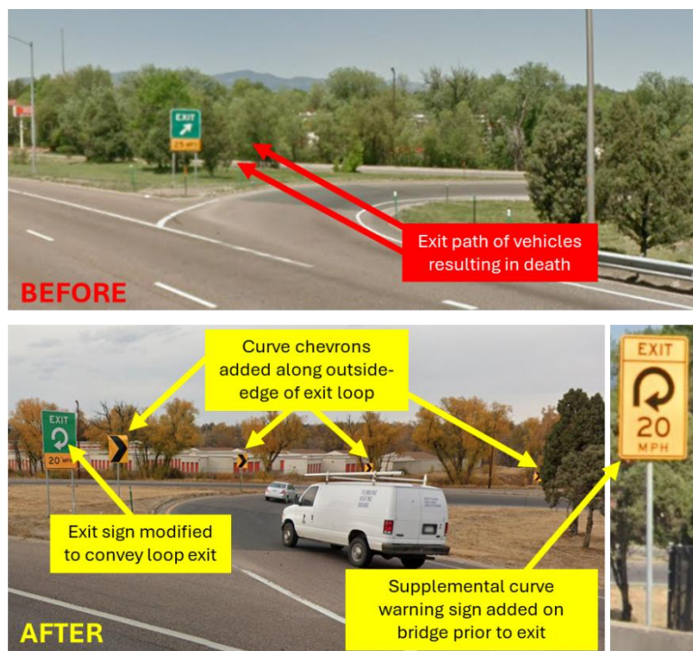
Exhibit 3: Example of visibility enhancements: The US6 westbound exit to SH121-Wadsworth Boulevard southbound was the site of three fatal nighttime motorcycle crashes, approximately one per year, where riders failed to navigate the curve and continued straight. In 2018, Lakewood proposed modified signage to CDOT, which was installed on the exit ramp. In the 5 years since, no further fatalities have occurred at this location.
